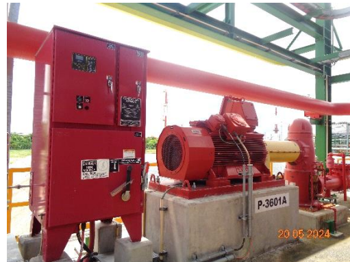
Electrical Driven Fire Water Pump
