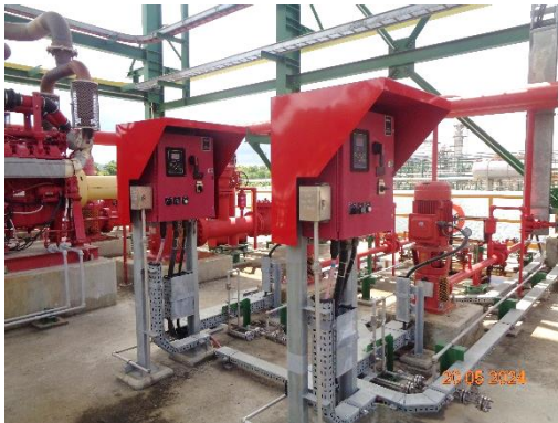
Electric Motor Driven Jockey Pumps
